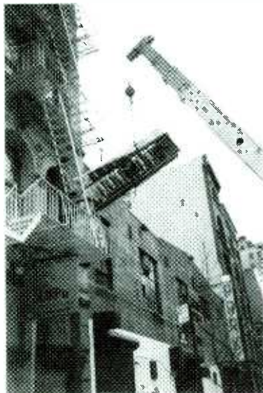
Kampo Cultural Center Studio takes delivery of an SSL 4056G console through a second-floor window—the only way it would fit.
